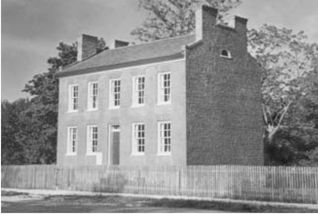
‘Api ‘o Uilifooti Utalafi ‘i Nāvuú
