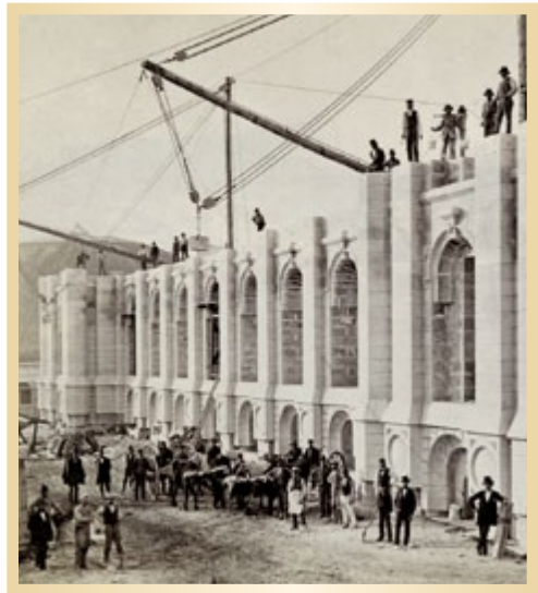
Construction du temple de Salt Lake City, 1877
