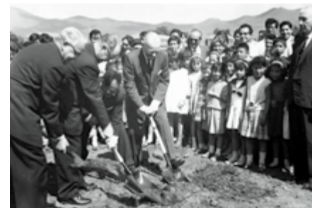
Church leaders participate in the groundbreaking for Benemérito de las Américas on November 4, 1963.
